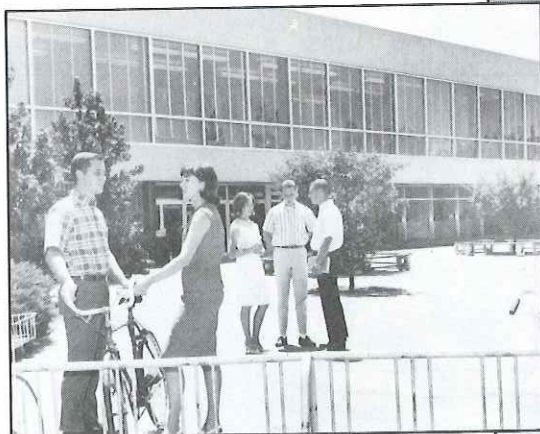
The newly constructed library on the Shaw Avenue campus was completed in December 1955. The library was named after Dr. Henry M. Madden, Fresno State librarian (1949-79), on October 11, 1981.
