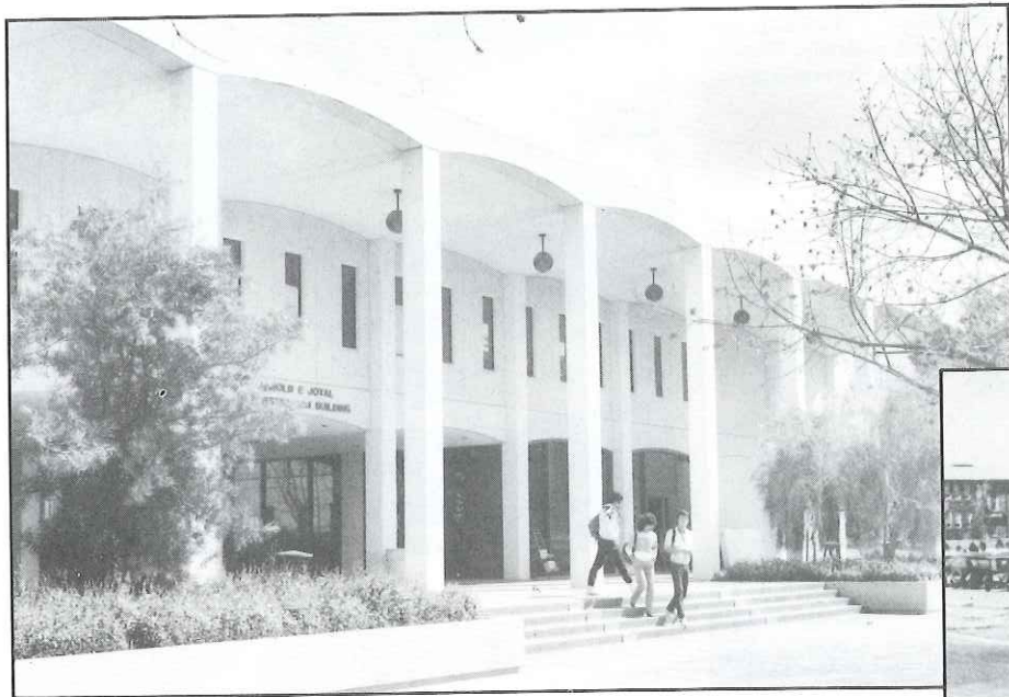
Joyal Administration Building, named after Arnold E. Joyal, the university's third president (1948-64), was completed in November 1967.
